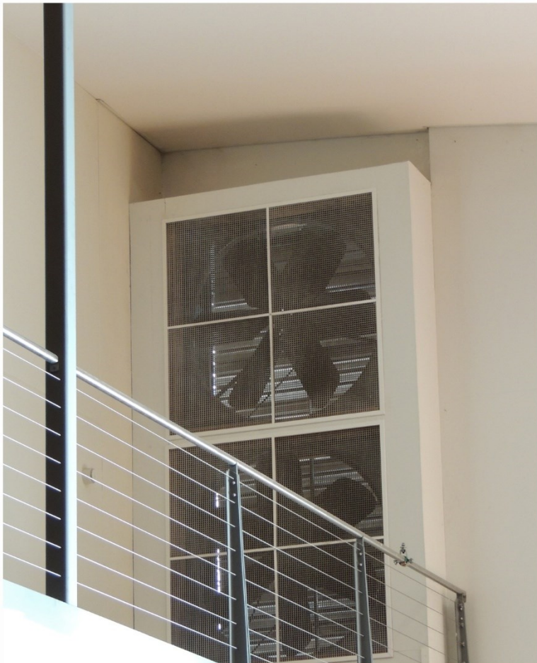
Whole House Fan Cooling System showing the ceiling shutter installed in the central stairwell of a two storey home.
