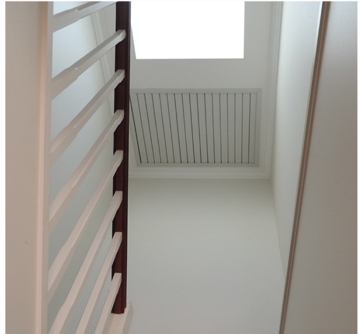
Whole House Fan Cooling System showing the ceiling shutter installed in the central stairwell of a two storey home.
